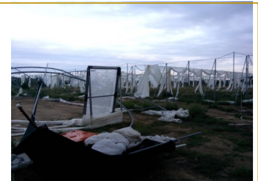
Damaged structures due to strong winds in an agricultural area (Miraflores) in Los Cabos, September 19 2014.
