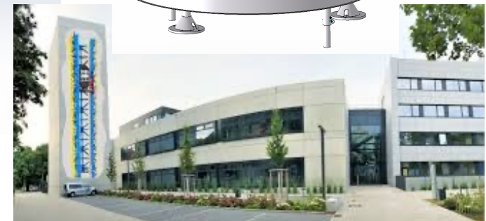
The Einstein Elevator Facility, Hannover, Germany 4 seconds of microgravity time, 100 shots a day
